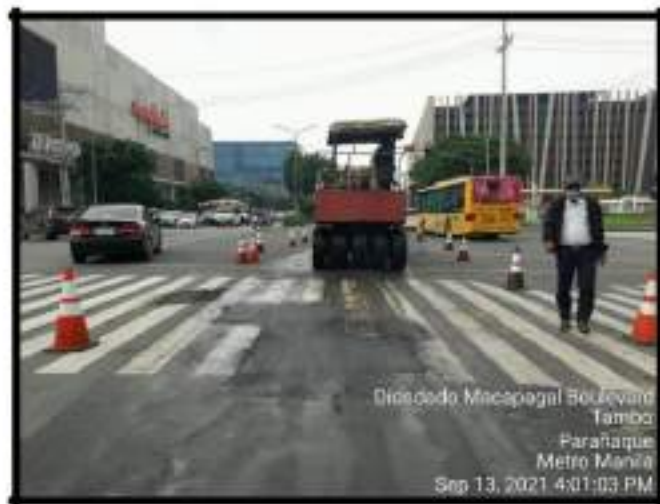
FROM NAIAX RAMP DOWN TO BELLE AVENUE
